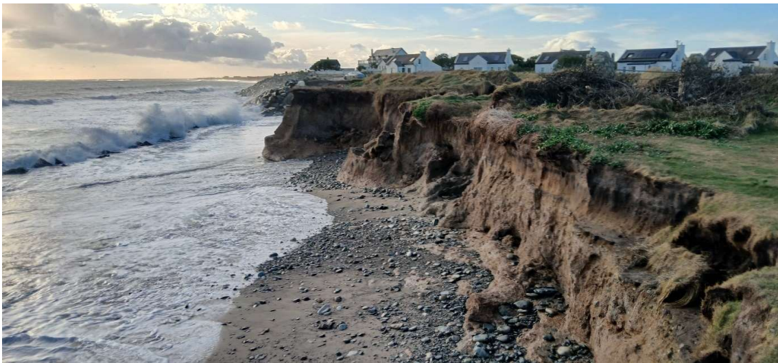
Coastal erosion at Seaview, Kilmore
