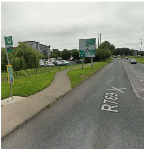
Newtown Road Scheme before works
