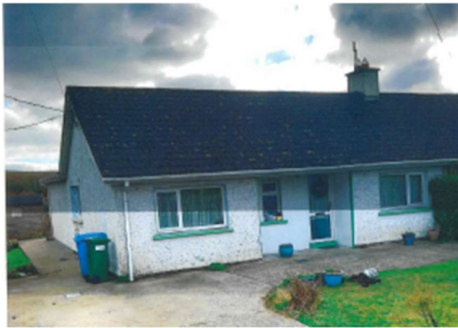
Property before Upgrade Works
