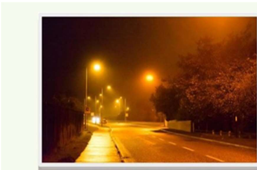
Photo of Public Lighting before LED Retrofitting
