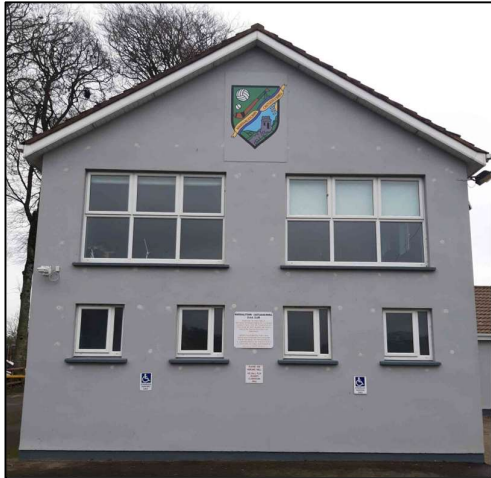
Cavity wall pumped at Marshalstown GAA Club
