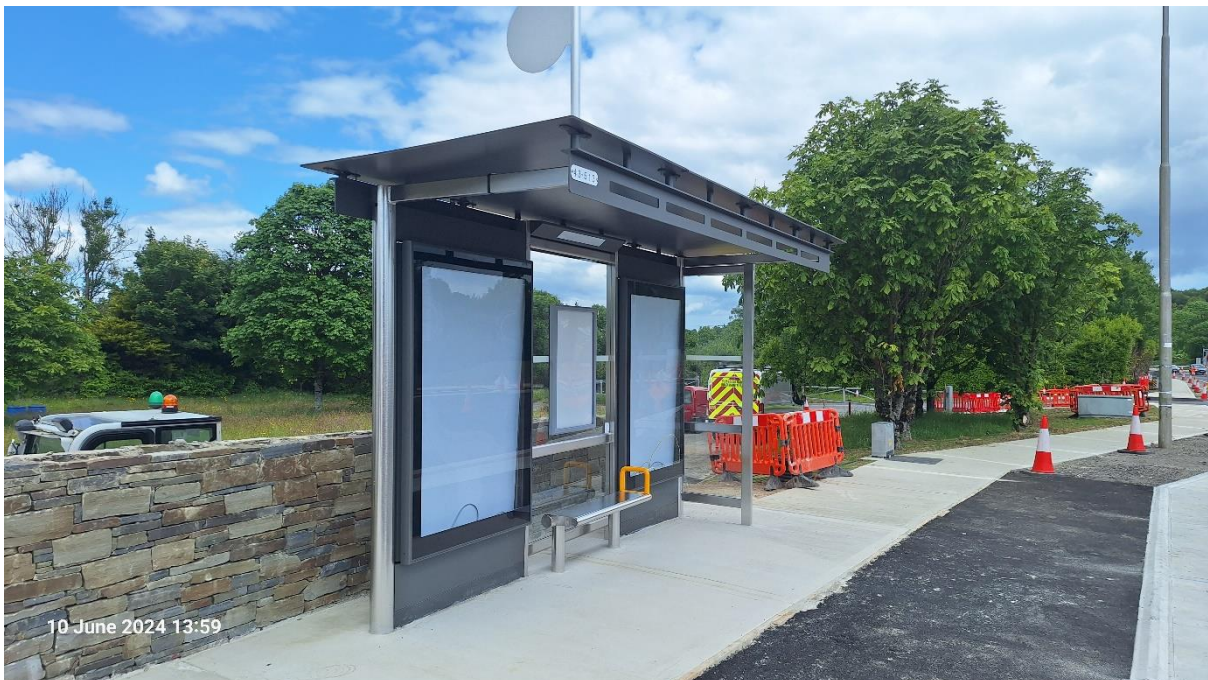
Fig. 1 Bus shelter installation Newtown Road
