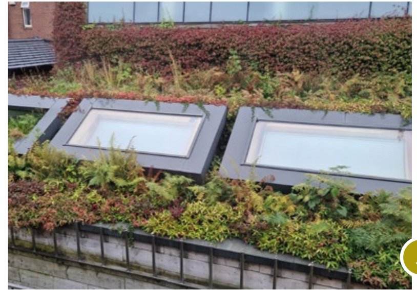
Figure 18: Green Roof - Engineers Ireland, Clyde Road, Dublin
