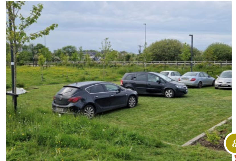
Figure 20: Proprietary Reinforced Grass - Min Ryan Park, Wexford
