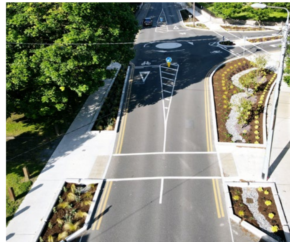
Figure 26: Carlow Raingardens (image courtesy of Carlow County Council)
