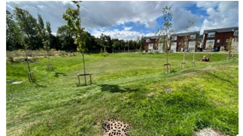
Figure 25: Detention Basin – Kilgobbin, Dublin
