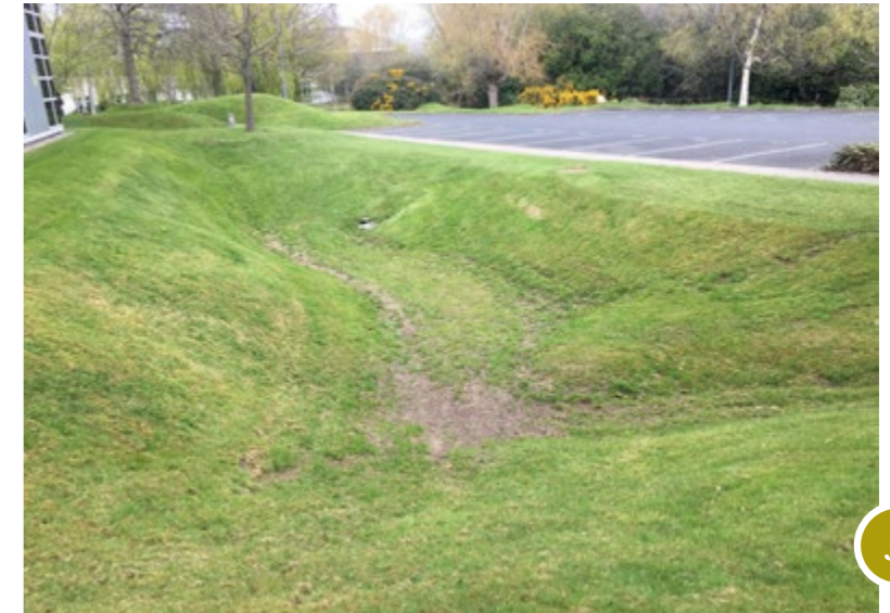
Figure 14: Detention Basin - City West, Dublin
