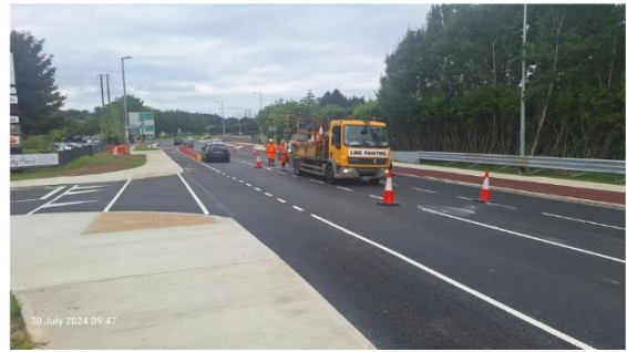
Fig. 3 Road markings being painted
