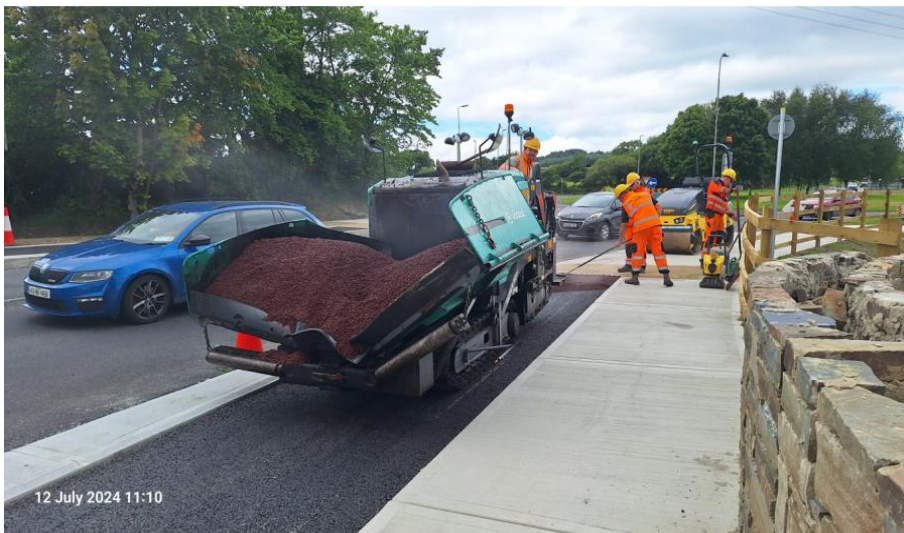
Fig. 1: Red surface being laid for cycletrack.
