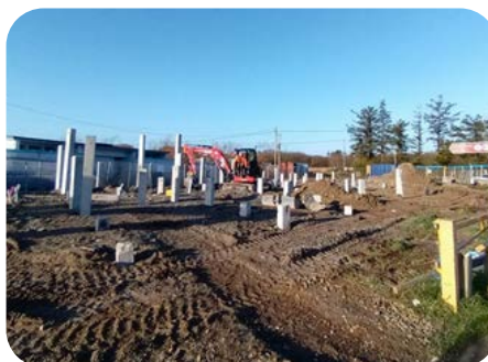
Curracloe Water Sports Activity Facility
