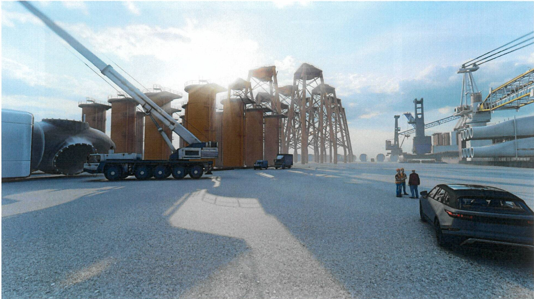
Figure 3-6: Example of Monopile and Jacket Foundations onsite for Offshore Wind Turbines
